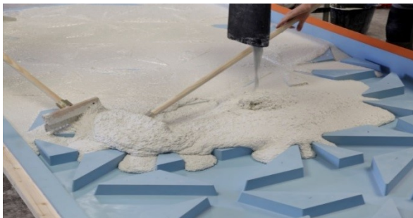
Figure 9: Concreting a prefabricated element
