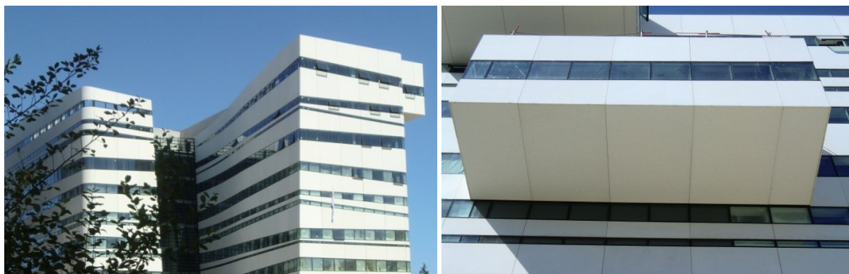
Figure 3: Dijon Regional Department of education (façade panels in white BSI®)
