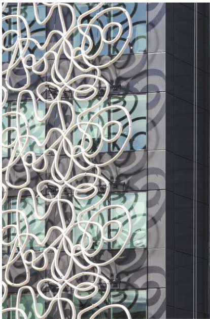
Figure 1: Ductal® lattice work panels- Vente Privée office, Saint-Denis (France) (©Atelier d'Architecture E. Nebout, ©photo Pierre Schwartz)
