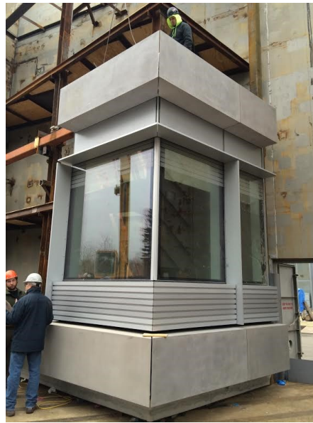
Figure 3: Full-size mock-up of the UHPC panel application for NYU's new Kimmel Pavilion
