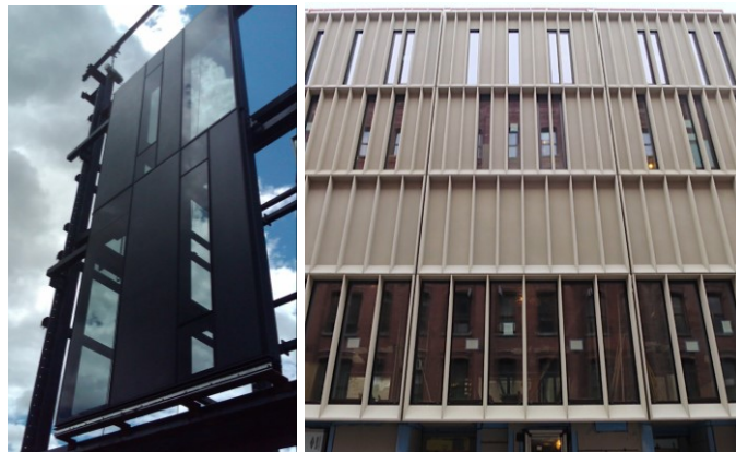
Photos 2: (left) Rotman Business School, Toronto, ON curtainwall w/ Ductal® UHPC flat panels and (right) Dumbo Lofts, Brooklyn, New York louvered rainscreen curtainwall [images Lafarge]
