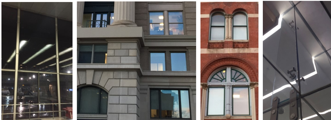
Photos 1: Steel, aluminum, stone, concrete, wood, brick clad and glass mullions [images Lafarge]
