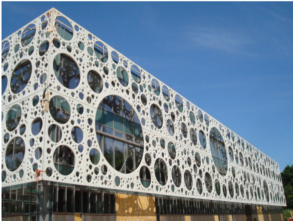
Figure 3: Installation of CRC façade elements for Odense University, Denmark.
