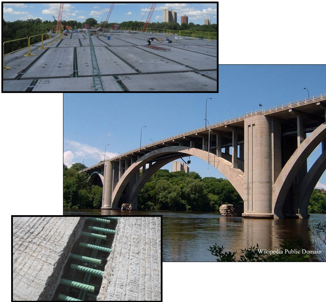
Figure 2: Accelerated replacement of the deck of the Franklin Avenue Bridge
