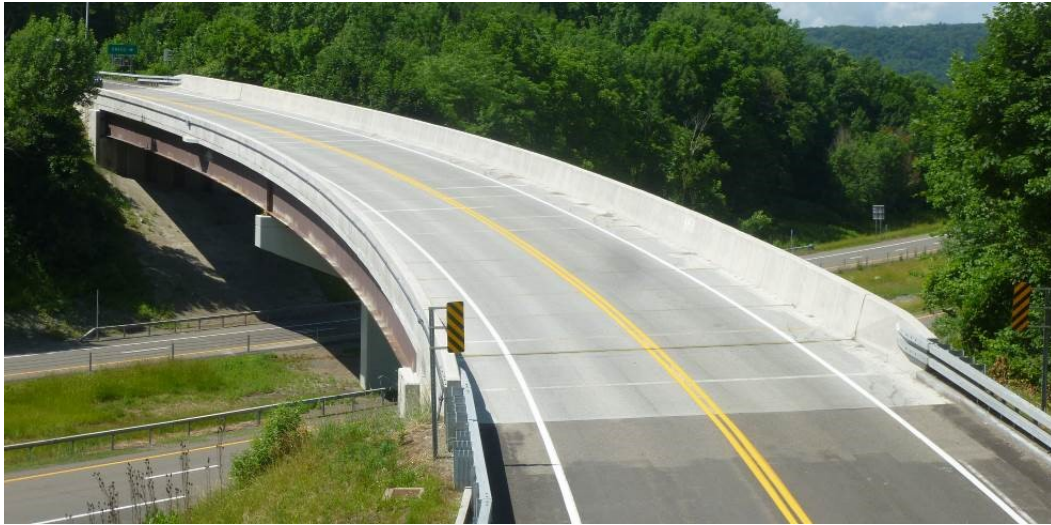
Figure 6: Bridge with UHPC deck level connections and a UHPC link slab (photo courtesy of New York State DOT)
