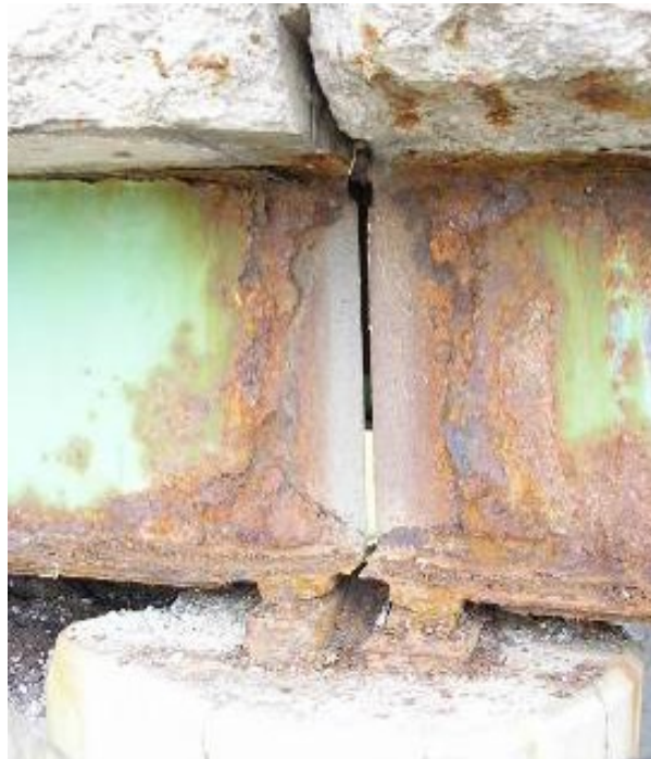
Figure 9: Deteriorated steel beams in need of repair (photo courtesy of New York State DOT)
