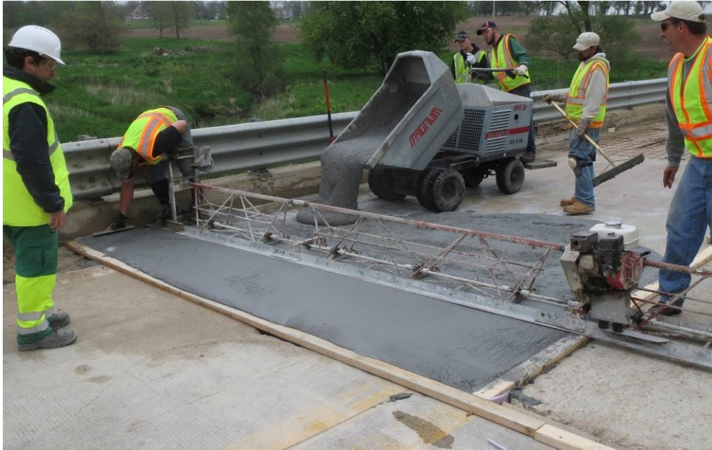
Figure 4: Installing a UHPC overlay to repair a deteriorated bridge deck
