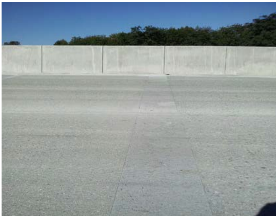
Figure 5: Finished Link Slab
