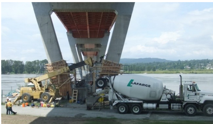
Figure 7: Batching & delivery to site by ready-mix trucks
