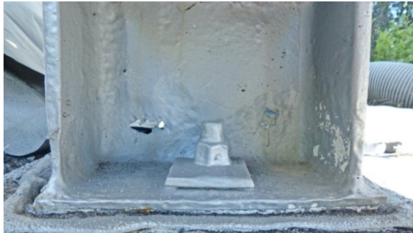
Figure 14: Corrosion at the base of a bent leg
