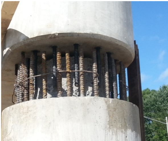
Figure 11: Existing rebar and new dowels
