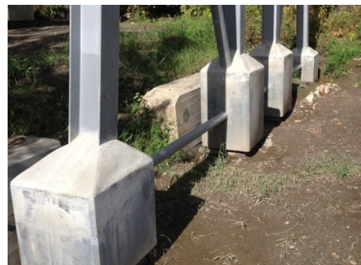
Figure 17: UHPC encasement of the bent leg bases after capping with non-shrink grout
