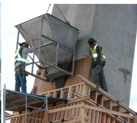
Figure 8: Placing via top of the form
