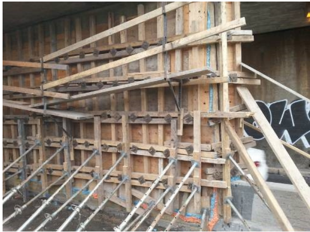
Figure 3: Formwork ready for casting
