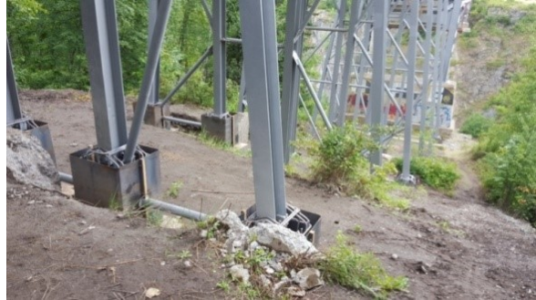
Figure 15: Bent legs with formwork for encasement
