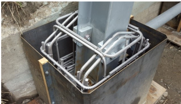
Figure 16: Reinforcing rebar cage and steel bolted to the flange leg
