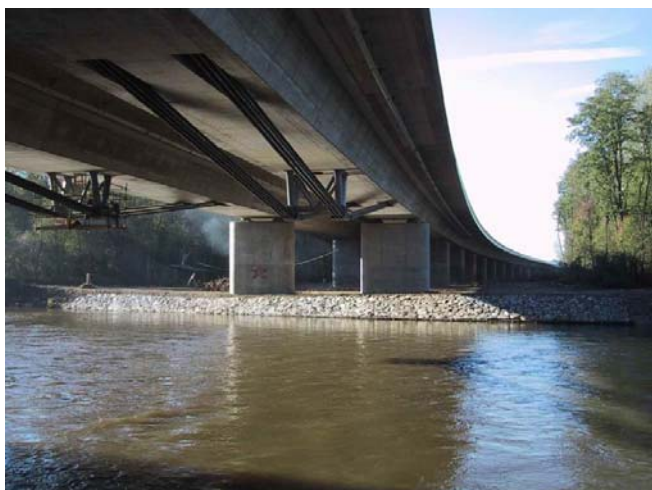
Fig. 11: Tendons under the structure
