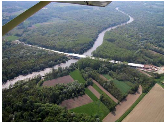
Fig. 10: The river, inundation zone and bridge during construction – May 2002
