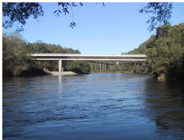
Fig. 12: The main span of the bridge
