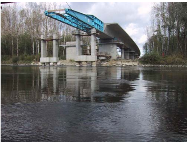
Fig. 9: Crossing the river with the first structure - November 2001
