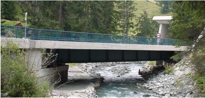
Fig. 7 Composite bridge strengthened by concrete overlay
