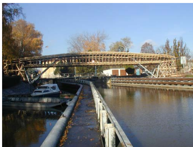
Fig. 9 Scaffolding and formwork
