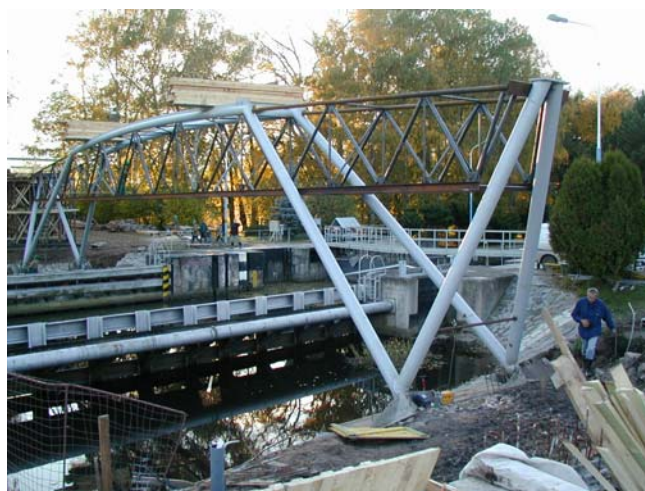
Fig. 5 Truss girder after erection
