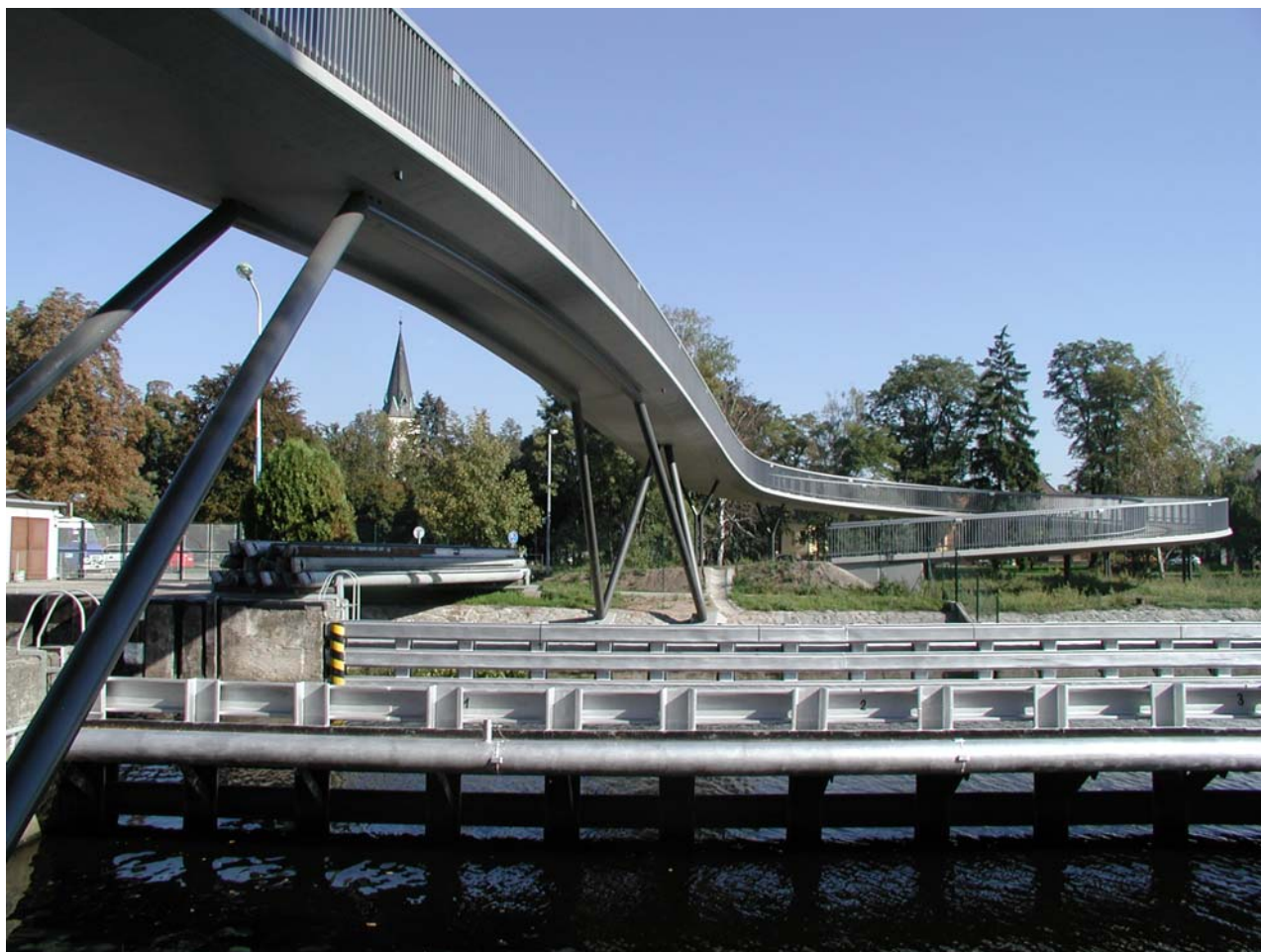
Fig.12 Play of simplicity - fluent curves of the concrete deck on the subtle steel supports
