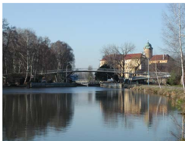
Fig. 8 The project completion in 12/2002
