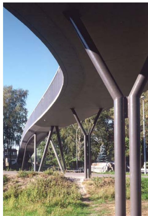
Fig. 4 The steel supports
