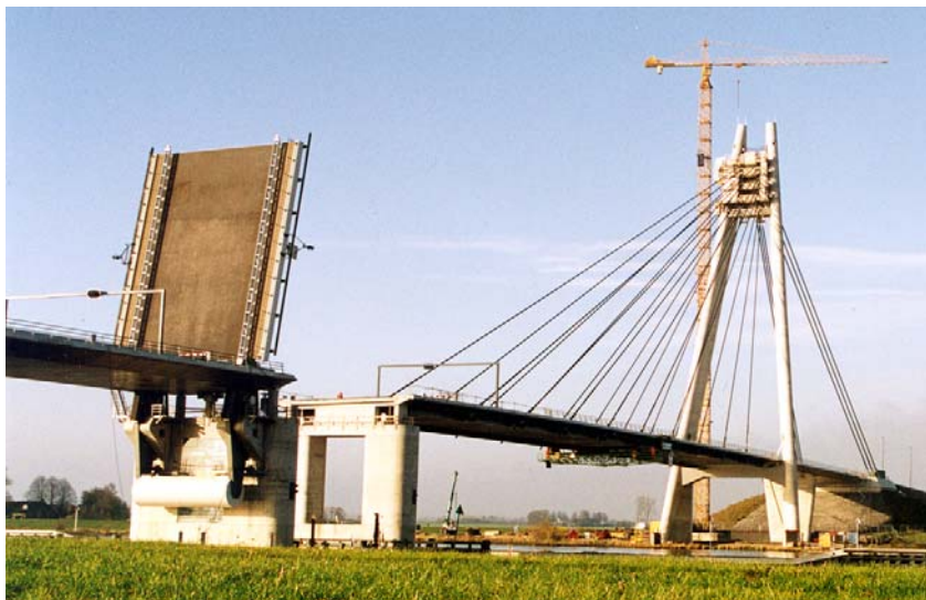
Fig. 2 Construction stage of a cable stayed bridge
