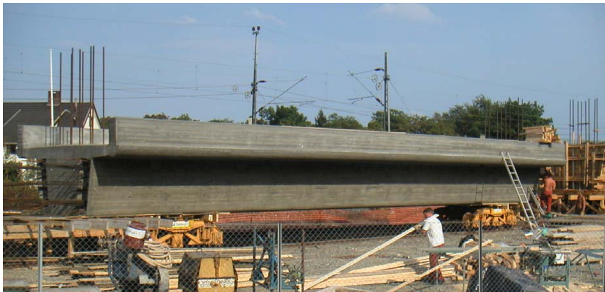
Fig. 4 Element 1 ready for transport to site
