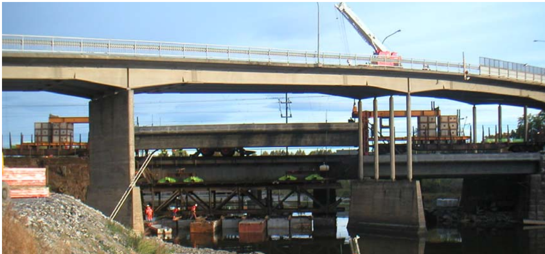
Fig. 6 Element 1 in position, ready to be lowered, existing steel truss cut down and lowered on pontoons
