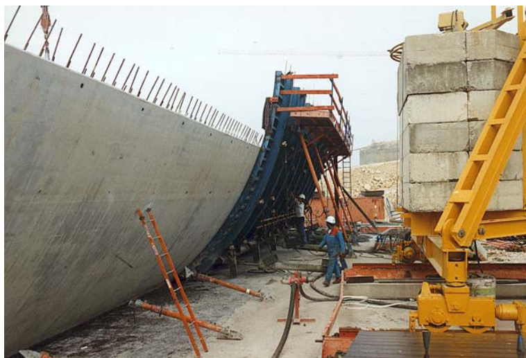
Fig. 3 Formworks on preproduction area
