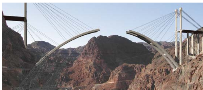
Fig. 8 Stayed Arch Erection
