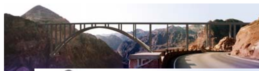
Short Span Concrete Arch with Composite Deck
