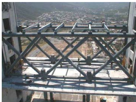
Fig. 4 Typical Steel truss
