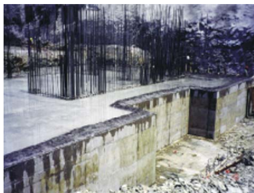
Fig. 7 Tower footing
