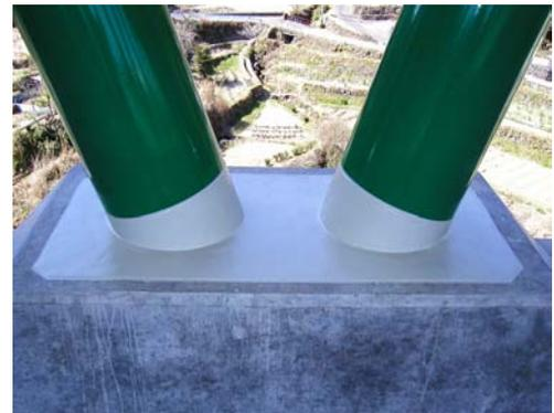
Photograph-4. Waterproofing coating
