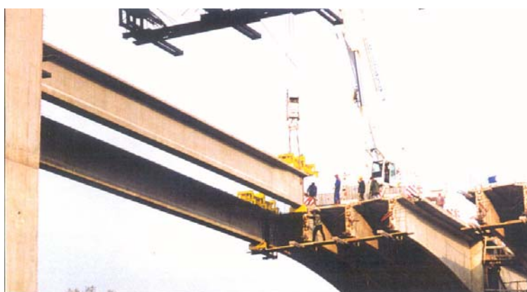
Fig. 8. Girder erection from river
