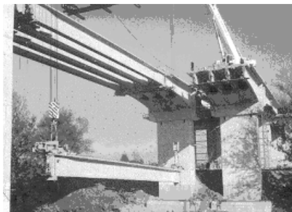
Figure 7: Girder placing at Kupa River
