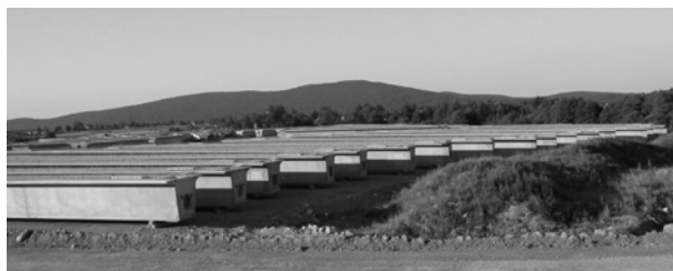
Figure 5: Girder storage at site
