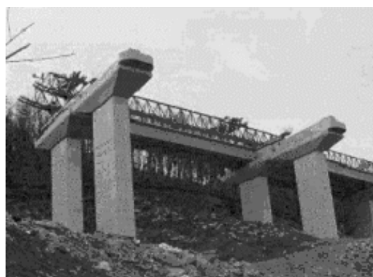
Figure 8: Girder launching – Viaduct Dreznik
