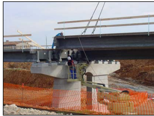
Fig. 5 Bourg-lès-Valence: erection of beams
