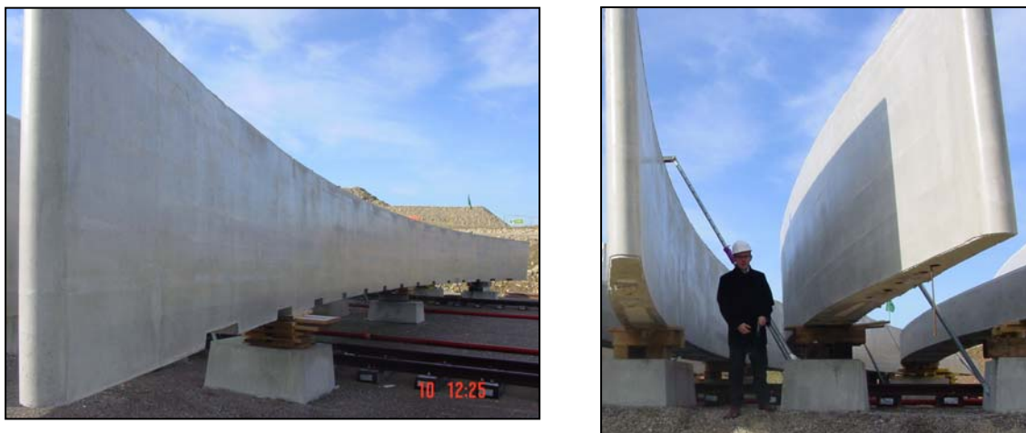
Fig. 15 & 16 Segments in storage yard awaiting installation on erection falsework
