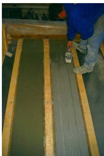
Fig. 8 Placing of the first layer of textile reinforcement
