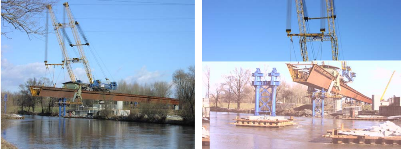
Fig. 23, 24 Odra Bridge - erection of the steel girder.
