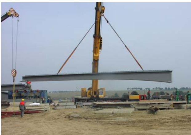
Fig.22 Overpass D216: erection of the plate girder
