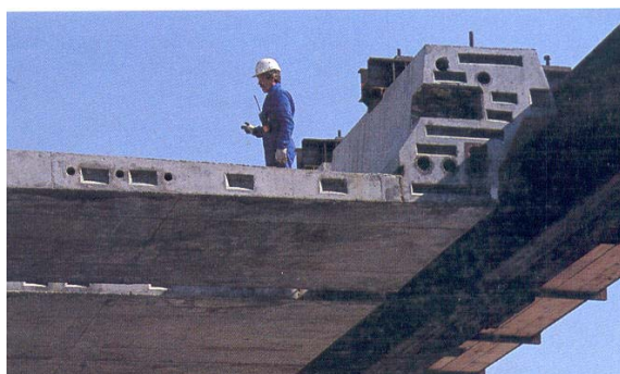
Fig. 2 Erection of segments using lateral support beams or under deck beams
