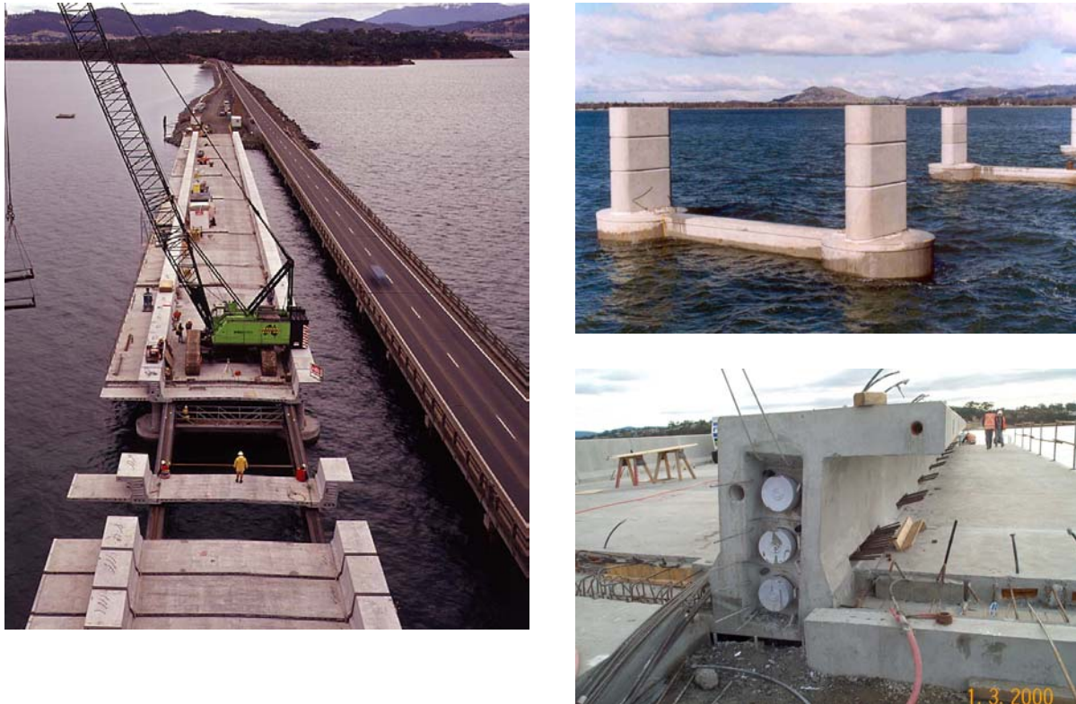
Fig. 4 Sorell Causeway Viaduct under construction in Tasmania, Australia
