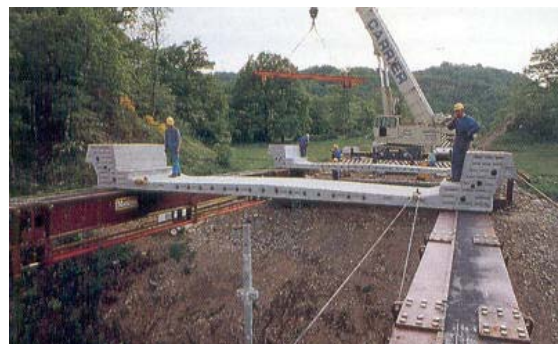
Fig. 2 Erection of segments using lateral support beams or under deck beams
