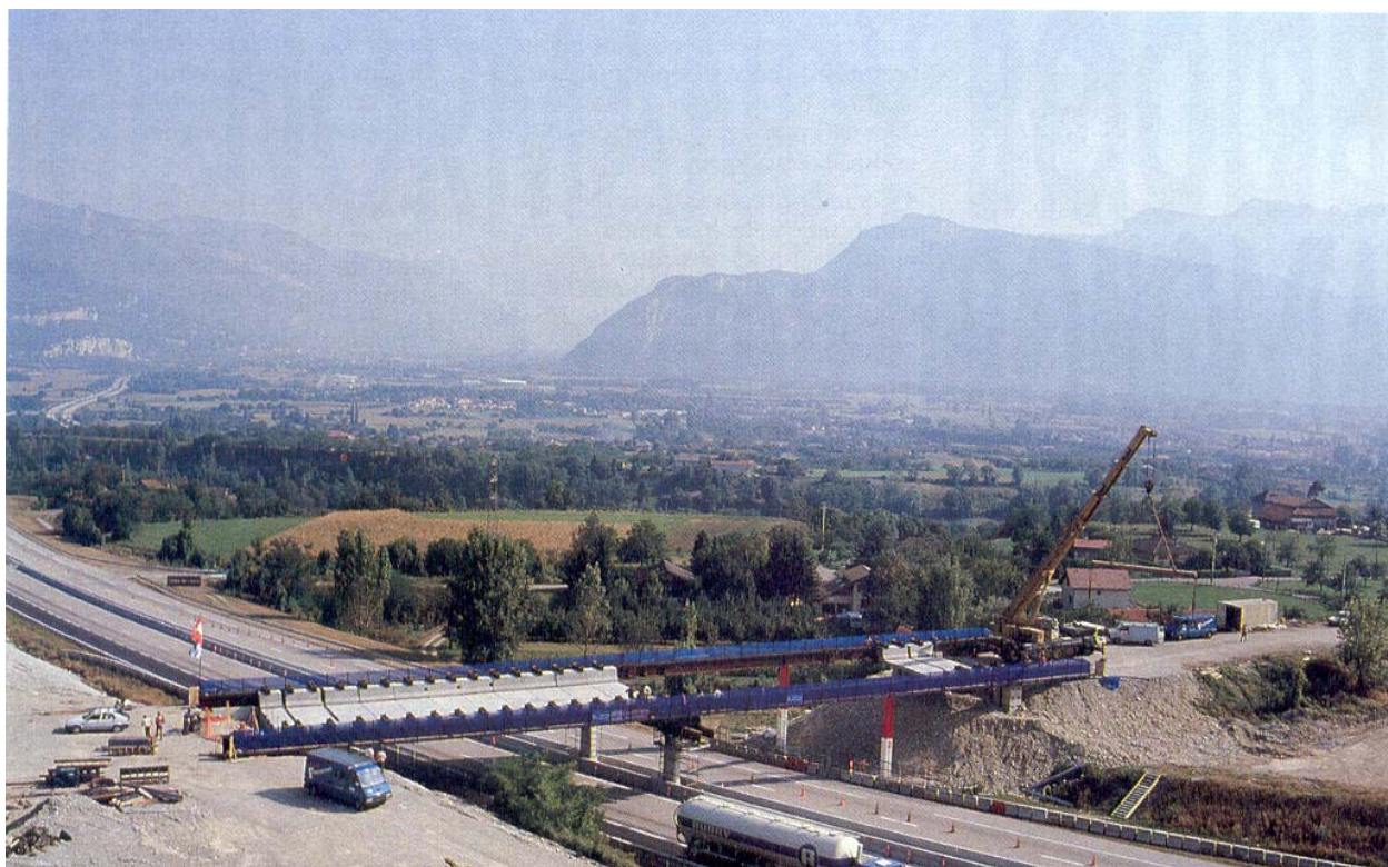
Fig. 1 The first channel bridge overpass under construction - Champfeulliet Overpass on the A48 in France
