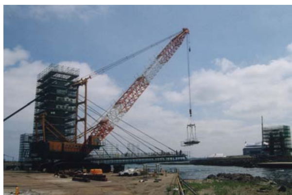
Fig.10 Erection of concrete segments
