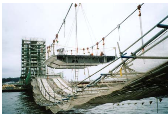
Fig.11 Erection of steel girders
