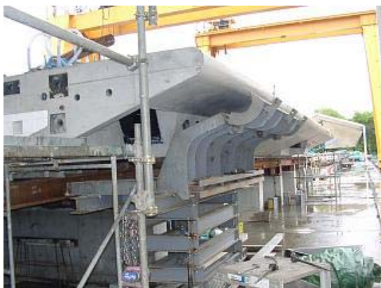
Fig.6 Fabrication of concrete segments
