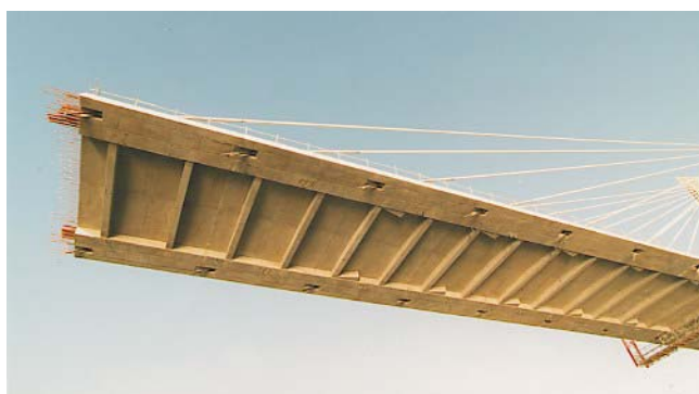
Fig. 7 Anchorage of stay cables under the deck
