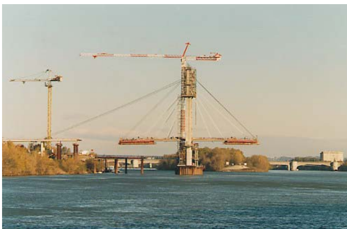
Fig. 9 Stability stays tensioned to balance the weight of the riverside segment
