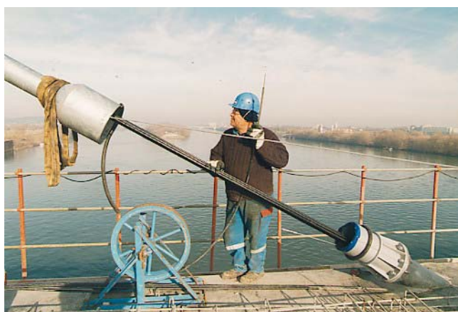
Fig. 6 Installation of the strands
