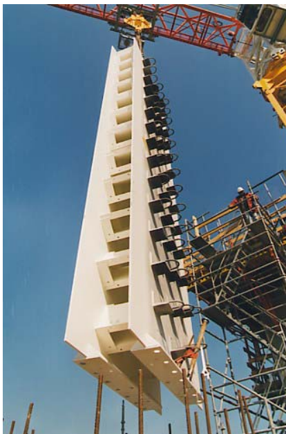
Fig. 8 Lifting of the steel anchorage box
