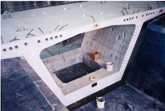
Fig. 5 Precast fixed bent segment
