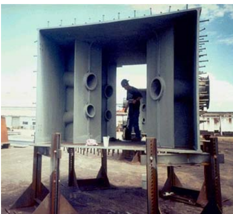
Fig. 11 Tower anchorage unit on its side
