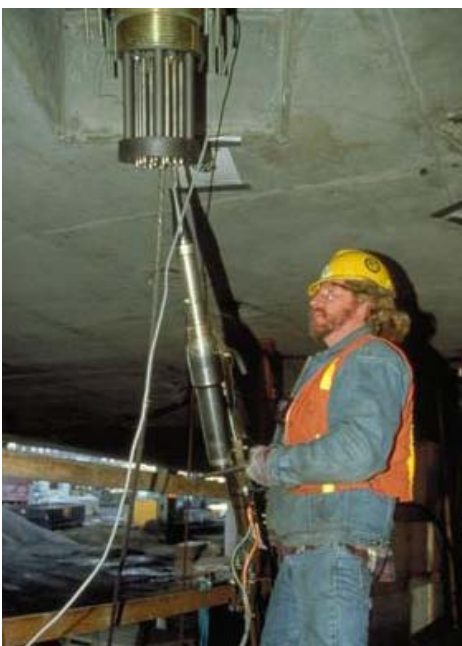
Fig. 12 Stay cable stressing, using “Iso-tension” method, in operation
