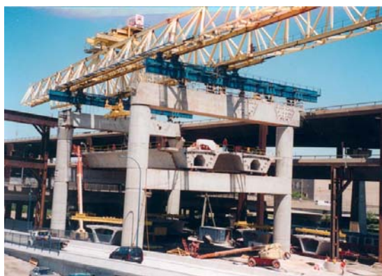
Fig. 4 Span-by-span erection at double-deck bents with overhead gantry
