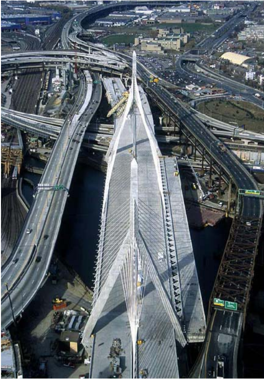
Fig. 9 Leonard P. Zakim Bunker Hill Bridge looking north, replacing the structure to its east
