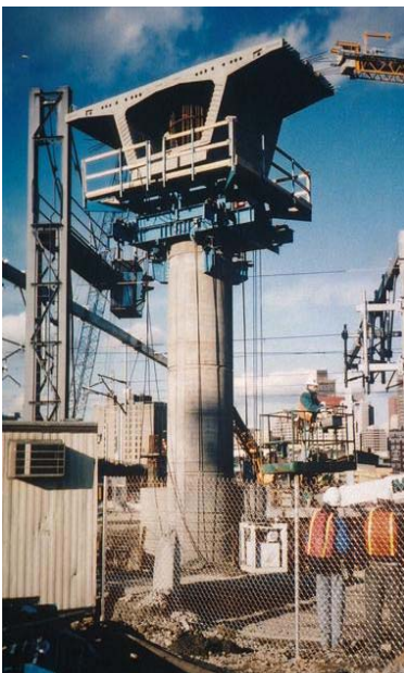
Fig. 6 Precast fixed segment in place on support frame
