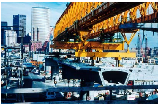
Fig. 3 Balanced cantilever erection using a gantry
