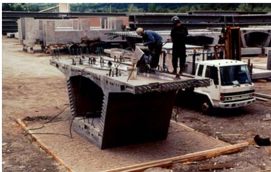
Fig. 7 Saw cutting of segment
