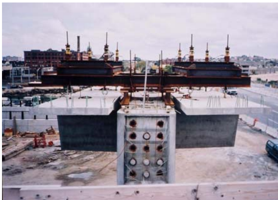
Fig. 8 Saw cut segments being erected
