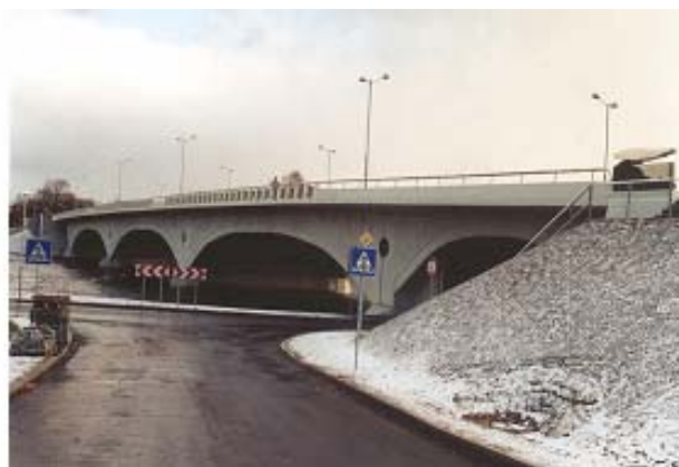
Fig.7 View on bridge after reconstruction
