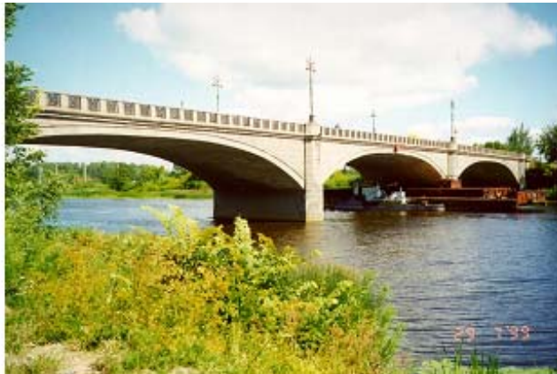
Fig.4 View on bridge before reconstruction
