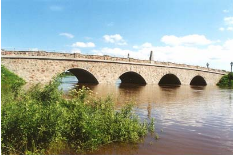
Fig.1 View on bridge facade
