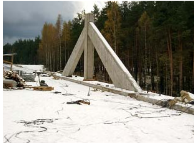
Fig.10 Overpass under construction
