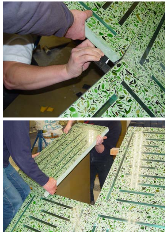
Fig. 7&8: The assembly of a small part of the dome with six panels with decorative glass strips in it.
