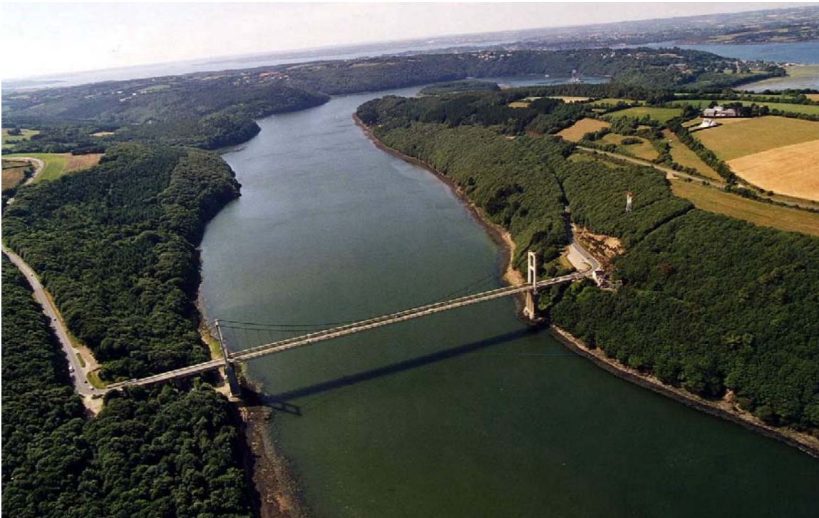
Figure 1 - View of the site and the existing bridge
