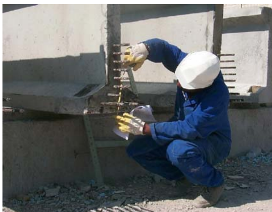
Fig. 2 Position of the protruding tendons
