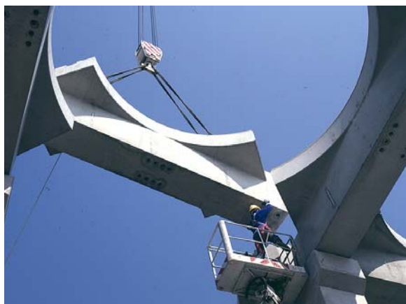
Fig.3 (a) Precast curved beams assemblage; (b) connection between the frame and the silos.
