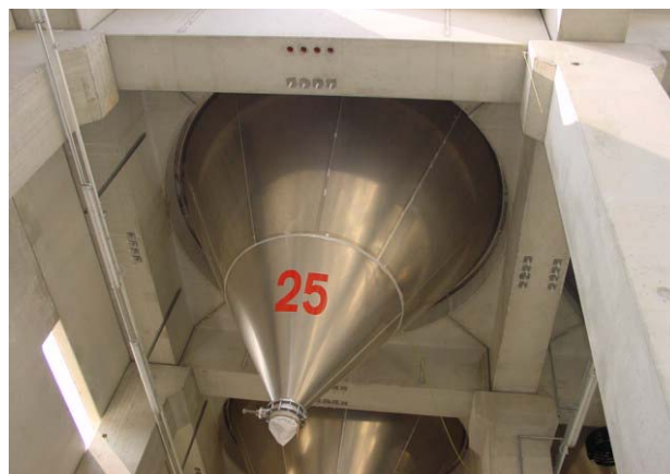
Fig.3 (a) Precast curved beams assemblage; (b) connection between the frame and the silos.
