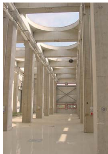
Fig. 4 Final frame ready for the housing of the silos.
