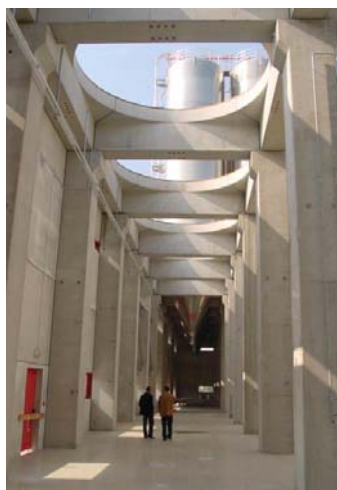
Fig. 4 Final frame ready for the housing of the silos.
