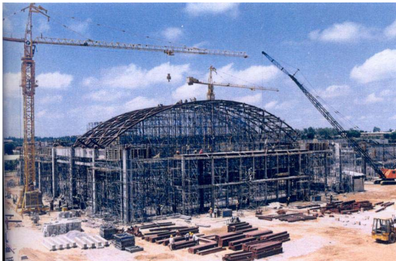
Fig.9: Erection of roof truss in progress
