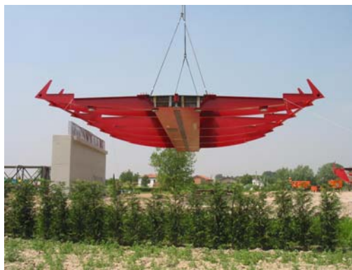
Fig. 8 : Bridge in Italy - Narrow box section with plate girder brackets
