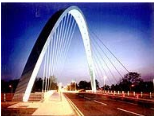
Fig.9: Hulme bridge, Manchester, UK.-50 m diagonal arch- 25 m high – bow section filled with concrete to withstand compression and bending( Phot Chris Wilkinson Architects)
