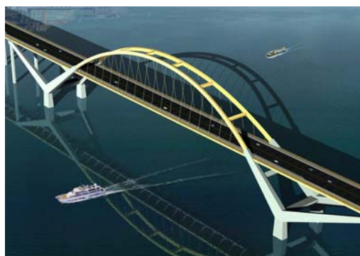
Fig. 10: Long span tied arch bridges : Caiyuanba bridge-China.420 m span,30 m wide; 6 road lanes and 2 walkways on upper deck, 2 monorail tracks on lower deck ( PhotoTy Lin International)
