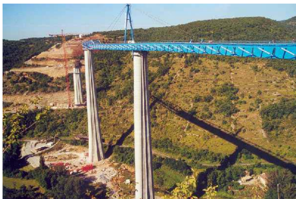
Fig. 7 : Verrières viaduct : Composite box section with inclined tubular brackets – 144 m amx span on 140 m high pier
