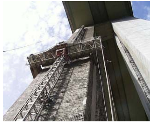
Fig. 2 Rehabilitation of the piles
