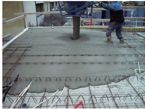
Fig. 2 Example of the use of Self Compacting Concrete at the casting of a bridge foundation and a slab of a house. No compaction is needed, improving the working environment and productivity.
