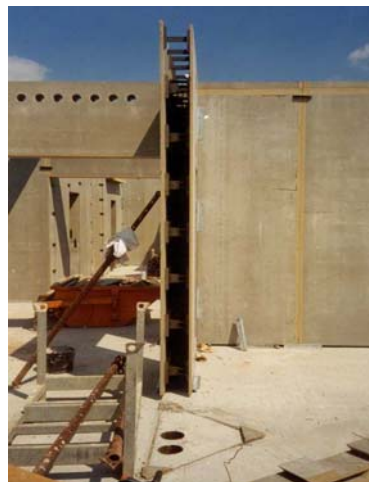
Fig. 3 The VS ® lightweight form system for effective construction with self compacting concrete.
