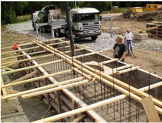
Fig. 2 Example of the use of Self Compacting Concrete at the casting of a bridge foundation and a slab of a house. No compaction is needed, improving the working environment and productivity.
