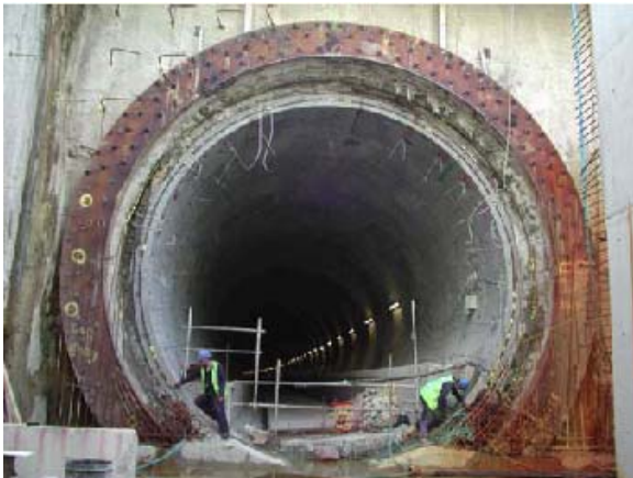
Fig. 3 Joint between TBM and Cut & Cover sections
