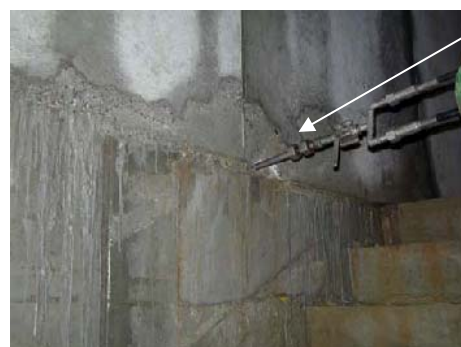
Fig. 13 Resin injection underway
