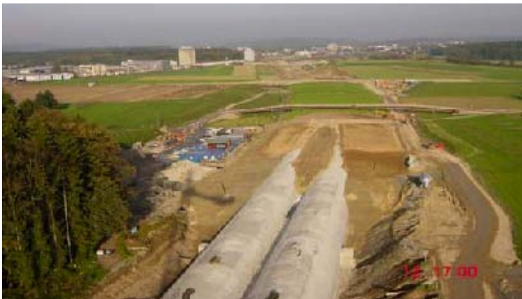
Fig. 6 Overview of Tunnel Thunstetten
