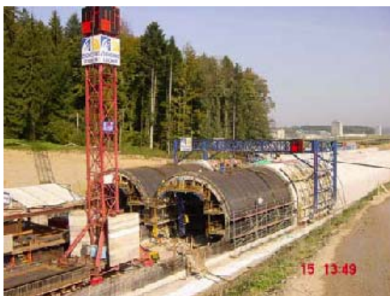
Fig. 7 Fixing steel and crack-inducer elements prior to concreting
