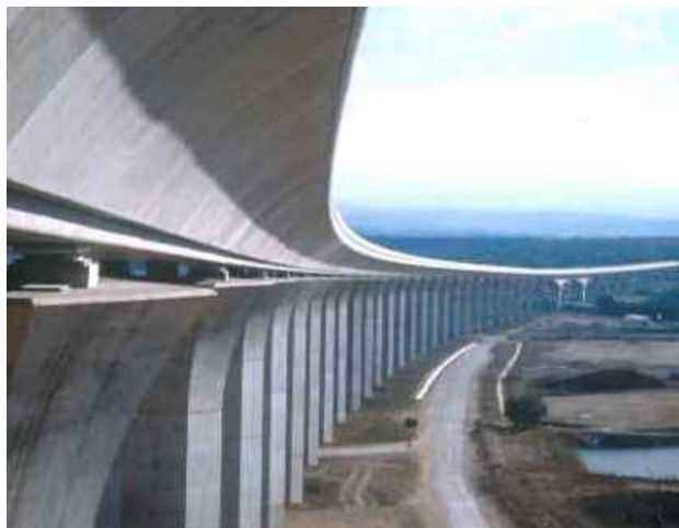
Fig 5. Viaduct of Ventabren
