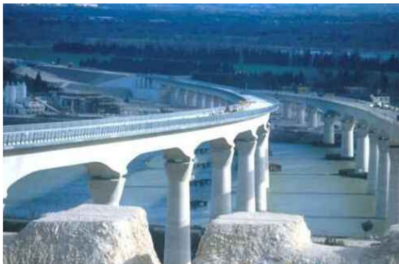
Fig 4. Viaduct of Avignon
