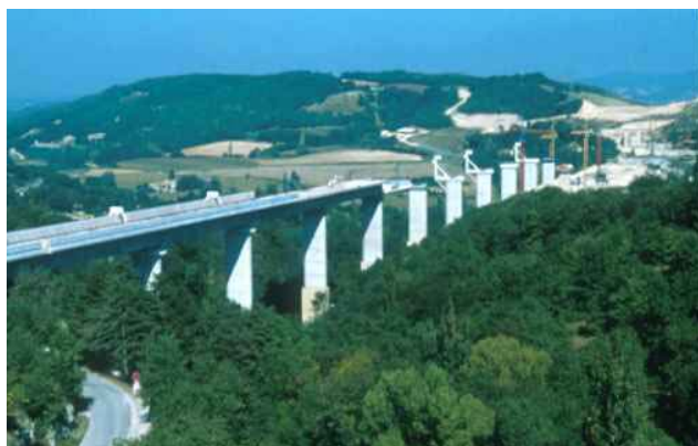
Fig 3. Viaduct of the Grenette
