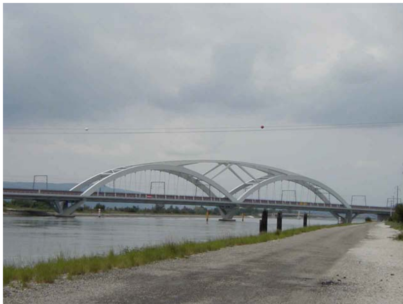
Fig 7. Viaduct of Donzère
