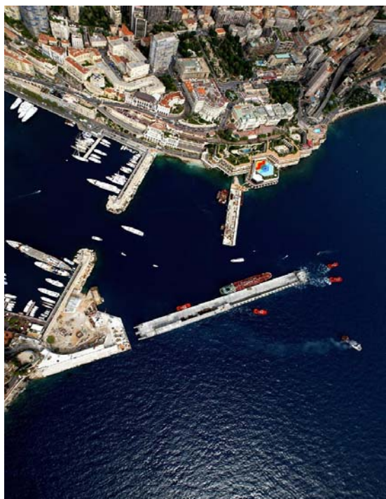
Final position of the dike prior to the installation manoeuvre
