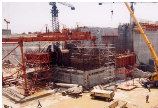
Encasement of the socket-and-ball joint
