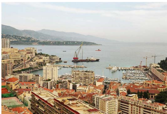
The 182m long crane ship driving piles inside the harbour
