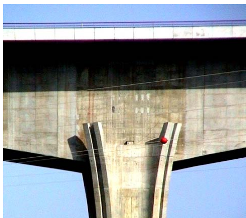
Fig. 25 Pier's connection with deck
