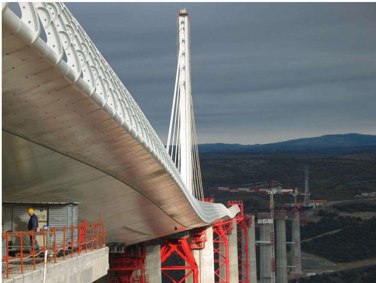
Photo 14: Deck during launching – south side
