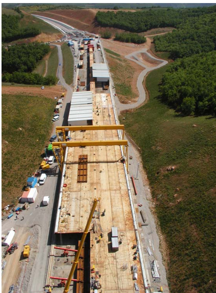
Photo 10: Area for prefabrication of the deck – south side
