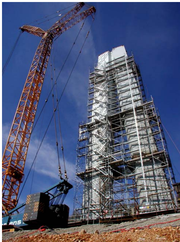
Photo 15: Lifting into position by crane of the elements of a launch pylon
