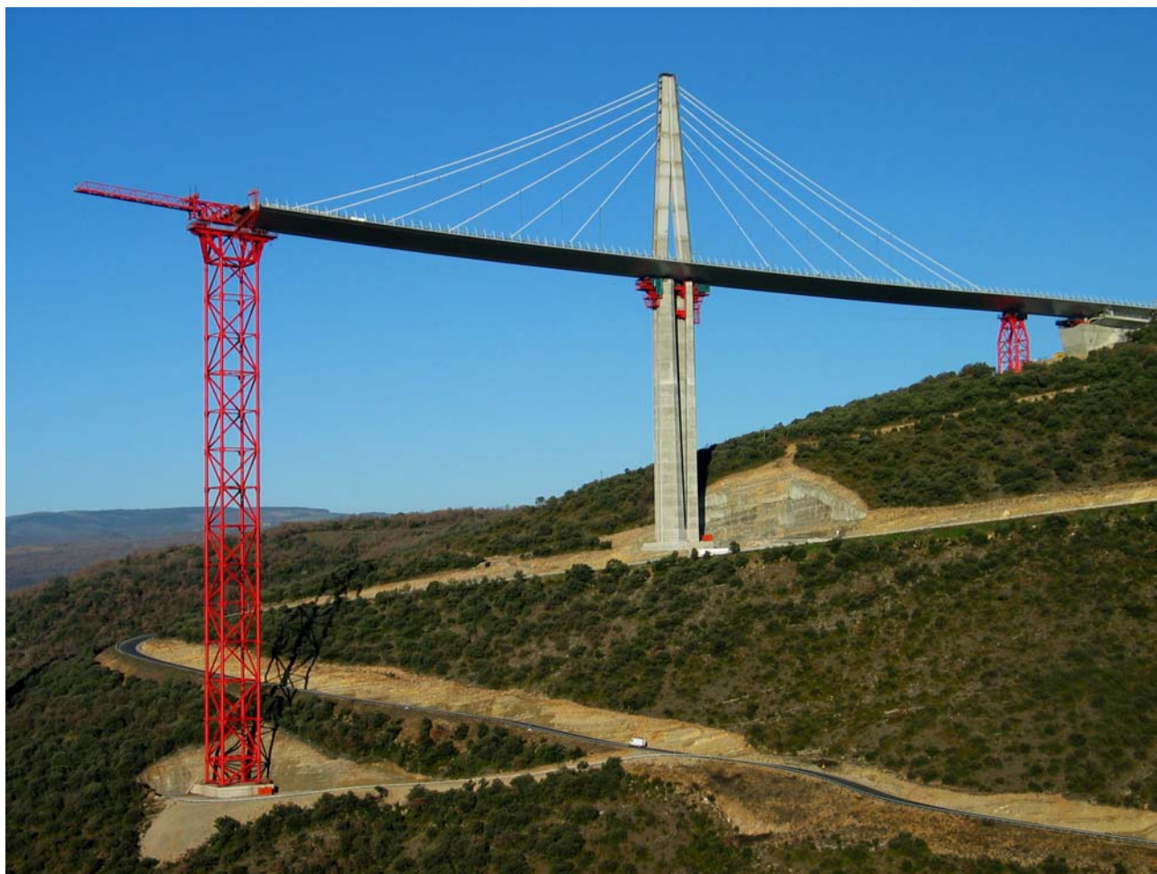
Photo 8: Docking of the deck on the temporary support Pi2 (height 173 m)
