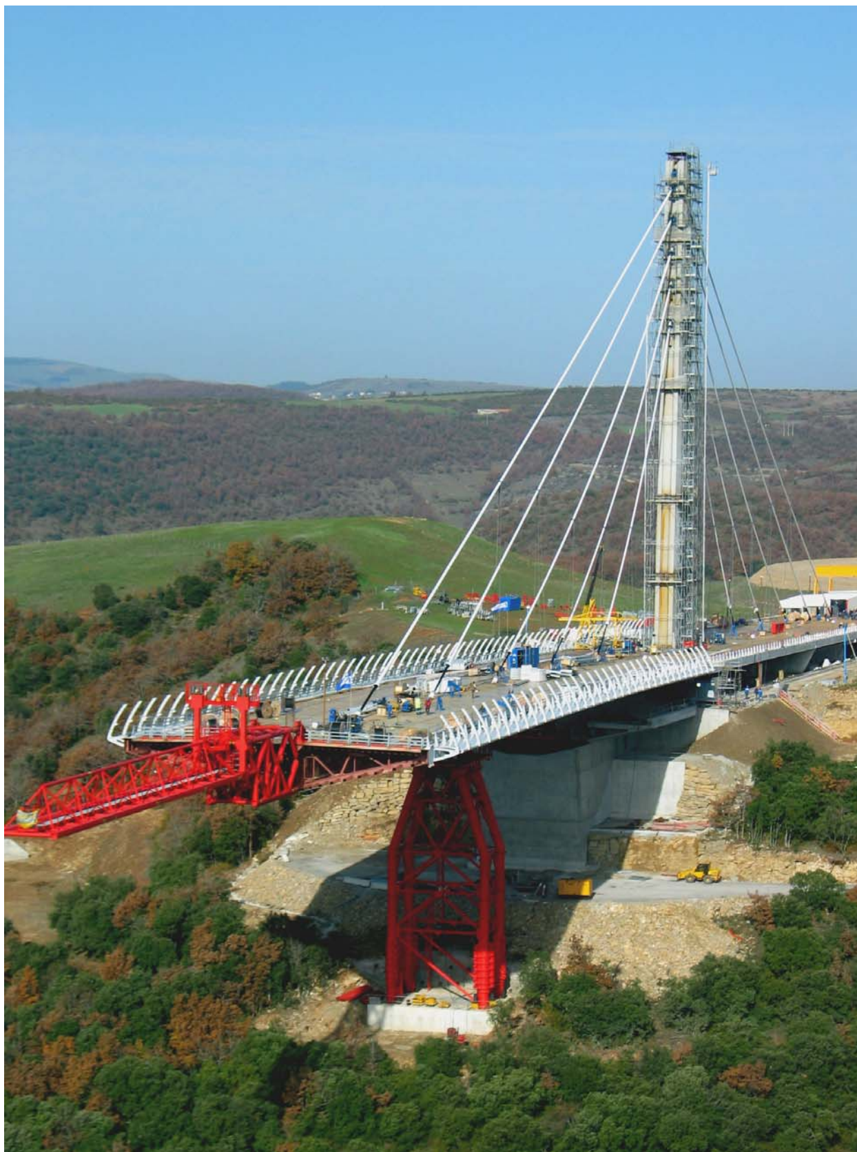
Photo 13: Nose fitted to the leading edge of the deck
