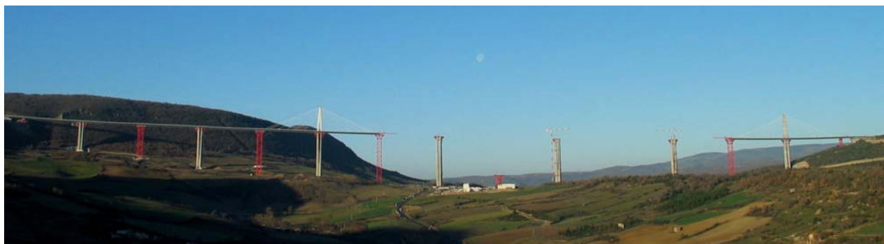
Photo 1: General view of the viaduct at the beginning of February after launches L8S and L4N
