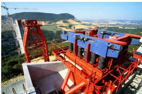
Photo 12: Deck launching system
