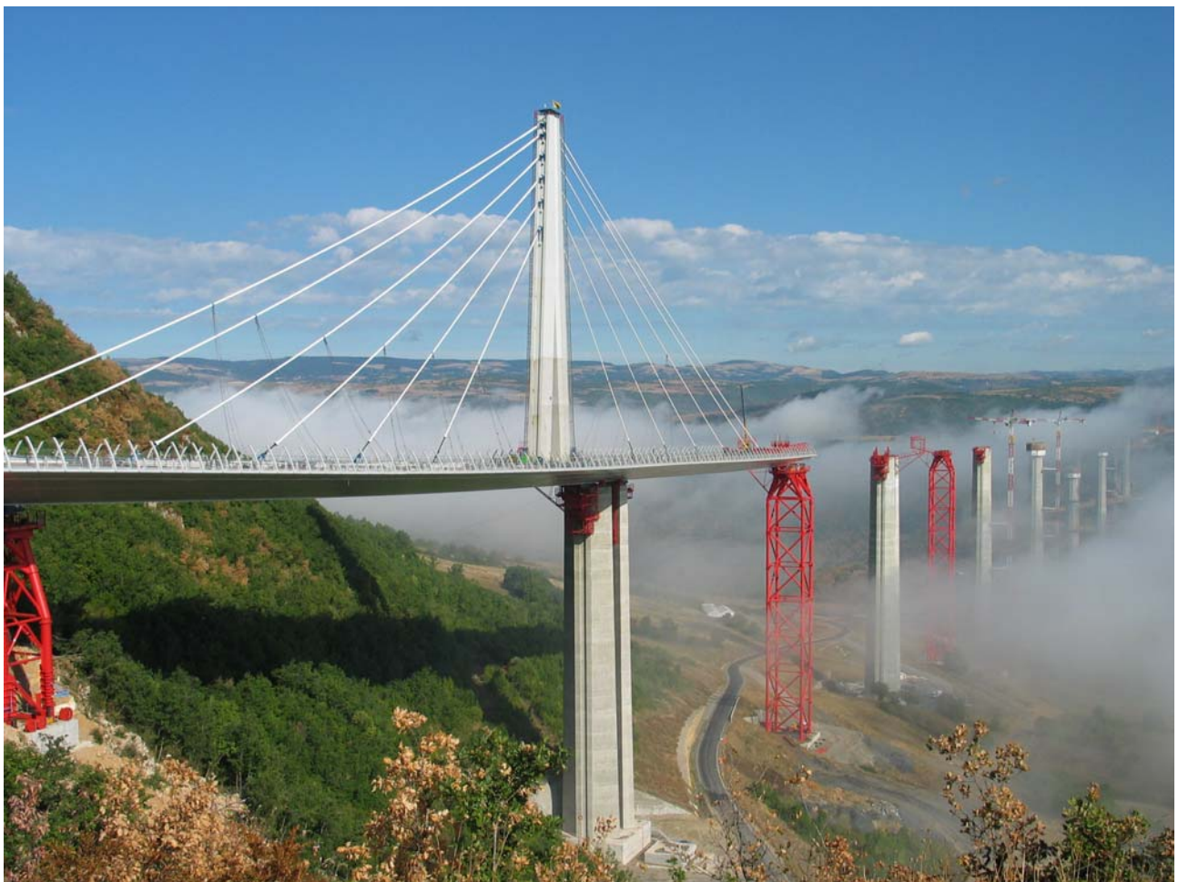
Photo 11: Launch L4S after re-tensioning of the stay cables
