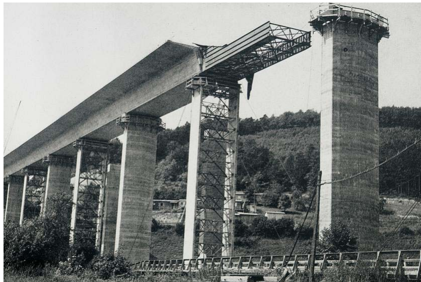
fig. 13: Incremental launching of a highway bridge
