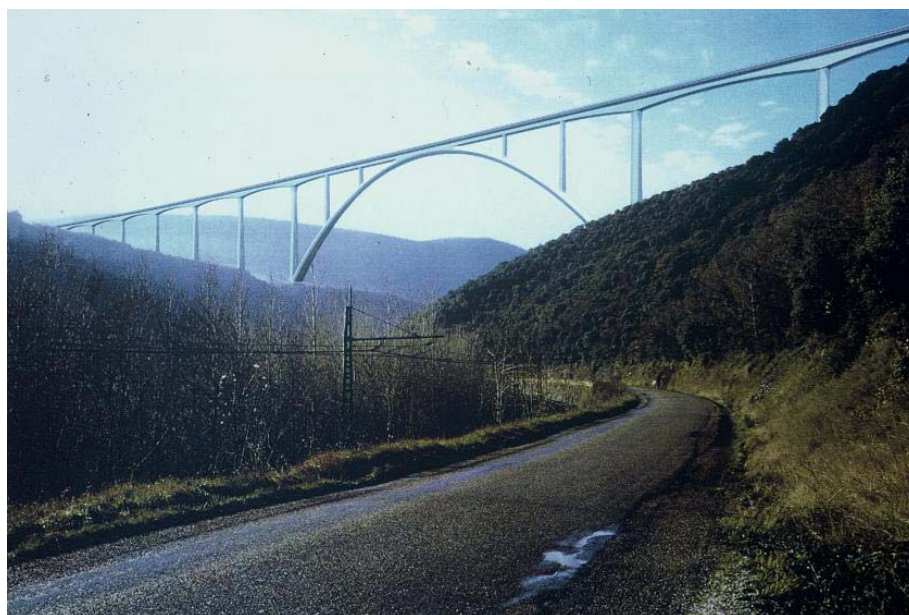
fig. 8: Proposal of an arch-bridge for the „Grand Viaduc de Millau“
