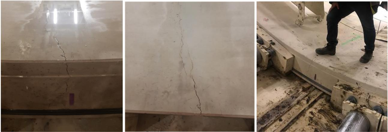
FIGURE 7 FISSURATION VOUSOIRS LOT 1 LIGNE 16 TBM6
