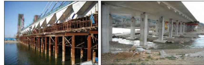
Figure 6.6: Concrete deck supported on temporary continuous or discrete propping
