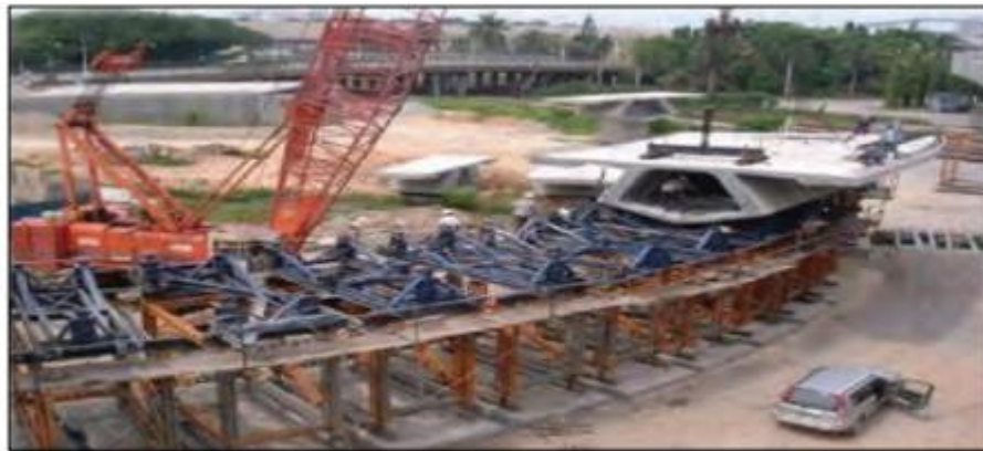
Figure 6.4: Erection of prefabricated segments on scaffolding
