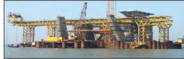
Figure 6.5: Erection of precast segments on scaffolding; all precast segments are lifted at one location by a lifting frame and slid on top of the scaffolding longitudinally
