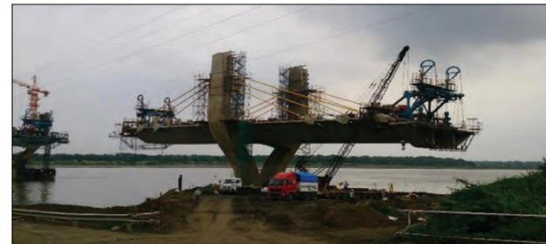
Figure 6.7: Balance cantilever technique
