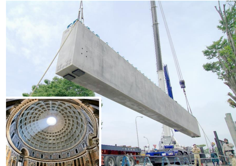
Zero Cement Concrete + Aramid FRP Tendons (2019)
