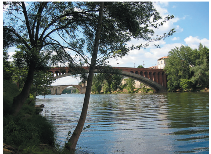
Pont de Villeneuve-sur-Loir © Association Freyssinet
