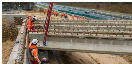
Figure 1. Placement of the reused bridge girders
