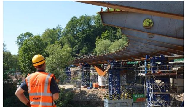
Figure 5. Temporary Launching equipment
